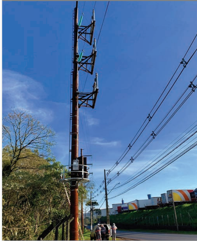
Figure 2. A side view of the Mark V Circuit-Switcher installation.
